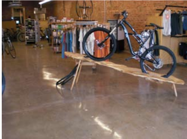
Polished concrete is as hard as Granite, reflects light well and is easily maintained.
